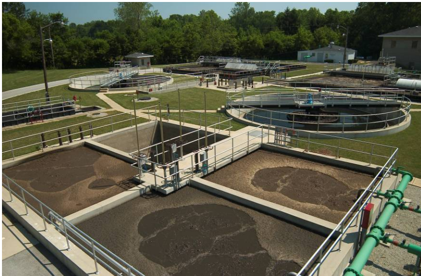
Inter-reactor tanks of Siemens' Cannibal installation at the Brookville WWTP.
